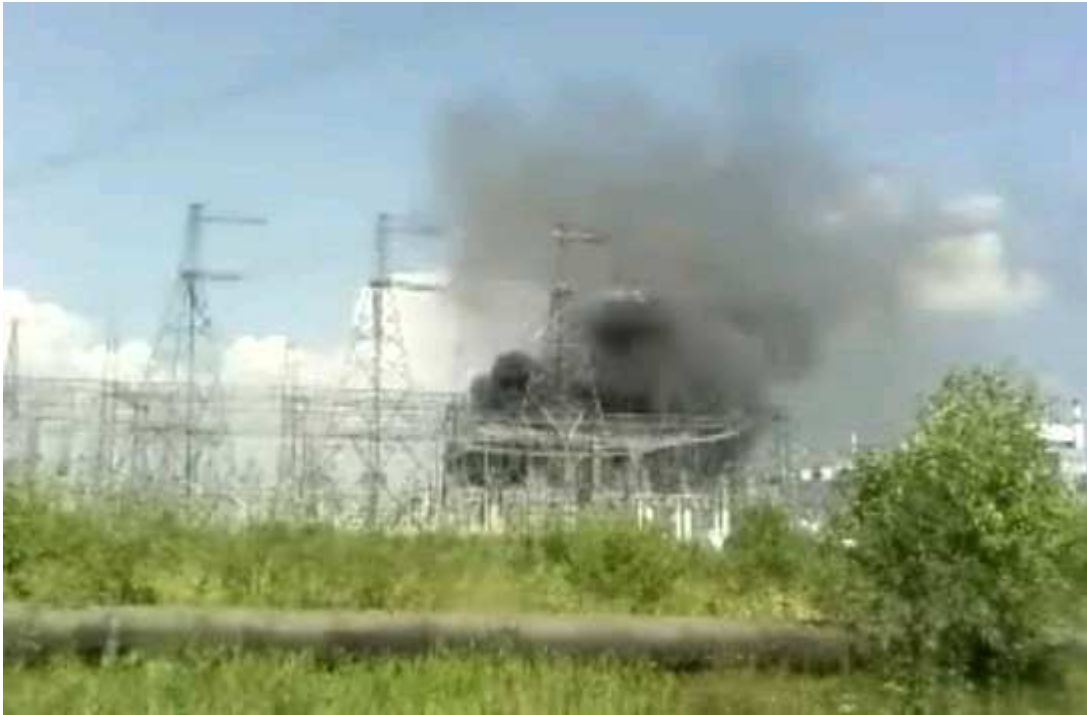
Image "Transformer fire atop the Kalinin NPP on June 23, 2010, Svetlana Zakharova » issue du site : http://www.bellona.org/articles/articles_2010/kalinin_repeats
